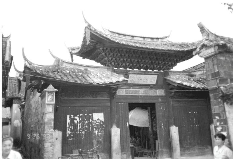
Fig. 5.3 (top) Watercolor of the Wuxi 浯溪 branch ancestral hall of the Miao lineage, Muyang village, from “Dong Lu Miao shi zongpu” (1936); and (bottom) the hall in 1997 (photograph by the author, 1997).
